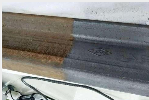
High-Speed Railway Track Rust Cleaning
